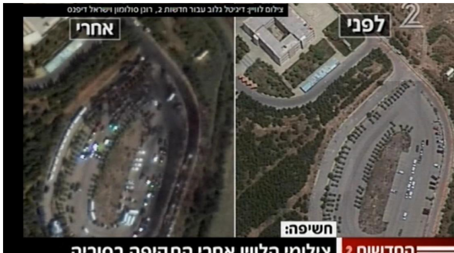
Image 1- A picture of the damage done to a parking lot at the Jamraya research center. The buildings appear to have been largely left intact [Aljazeera]
